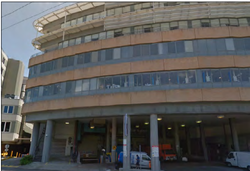
St. Vincent's Hospital along Boundary Street
